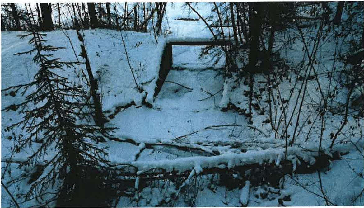
Photo 4 Downstream Side of Concrete Spillway Structure with Woody Debris in Outlet Channel
