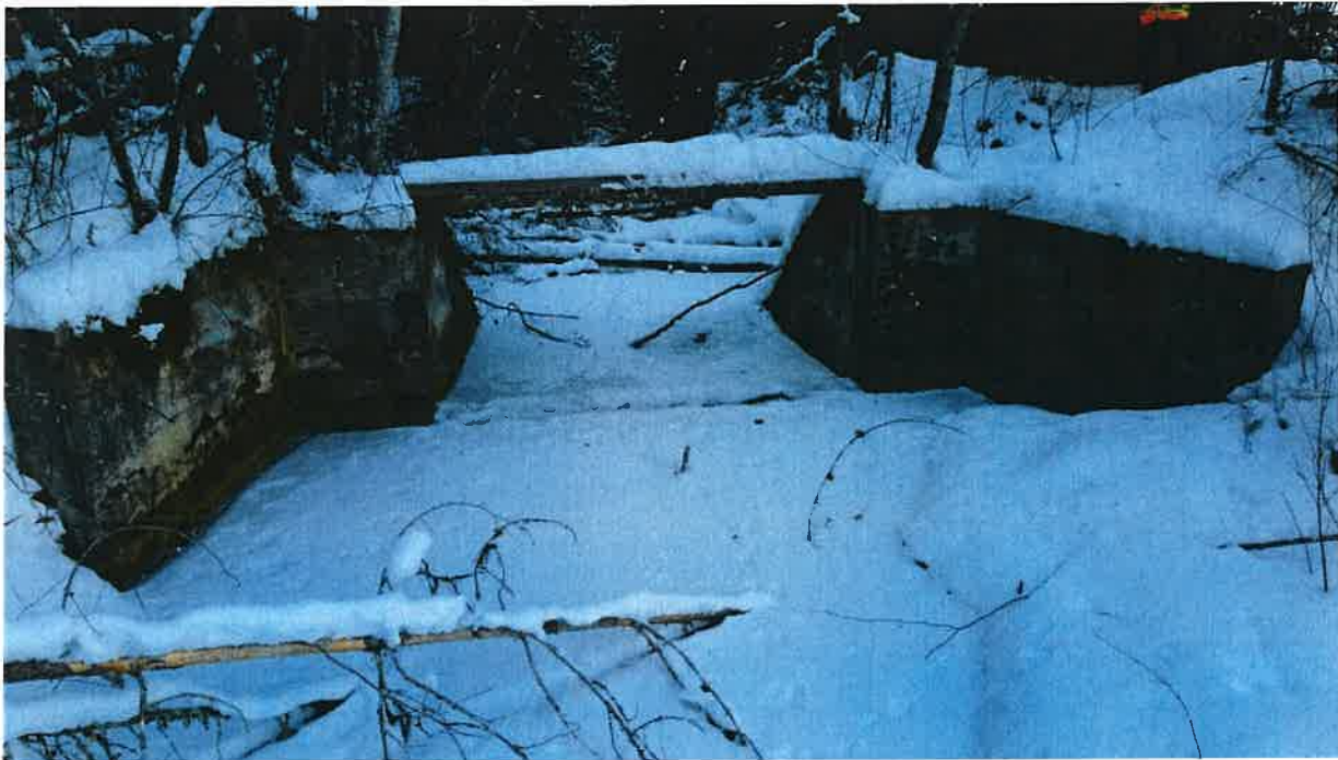
Photo 3 Upstream Side of Concrete Spillway Structure
