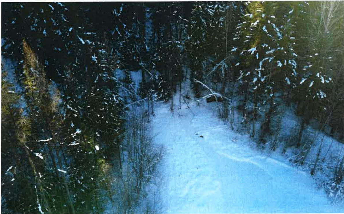
Photo 6 Frozen Spillway Inlet Channel
