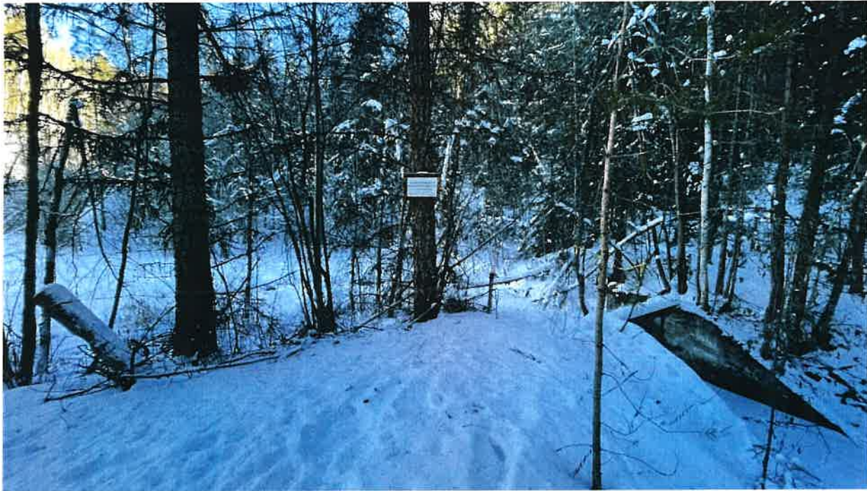
Photo 7 Emergency Signage Near Spillway Structure
