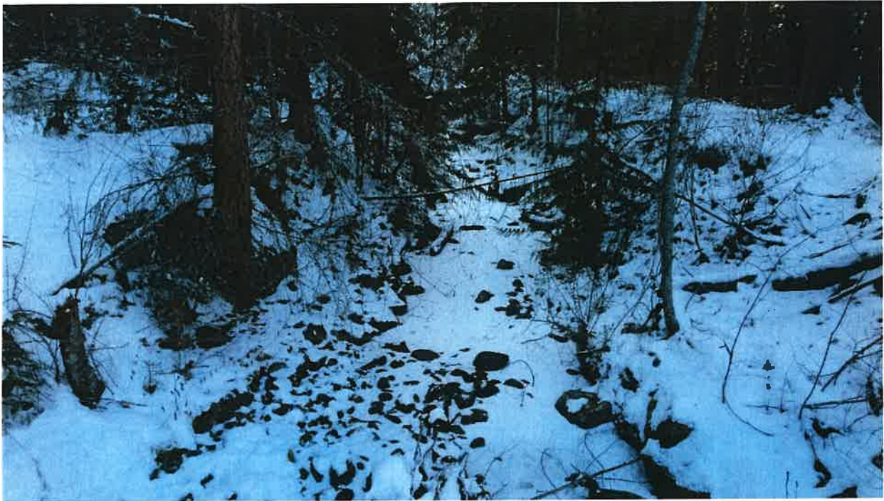
Photo 5 Spillway Outlet Channel with Ice
